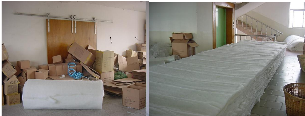
(Example: Obstructed emergency exits)
