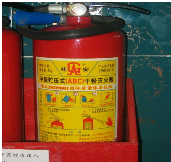
(Example: Fire extinguisher with instructions)
